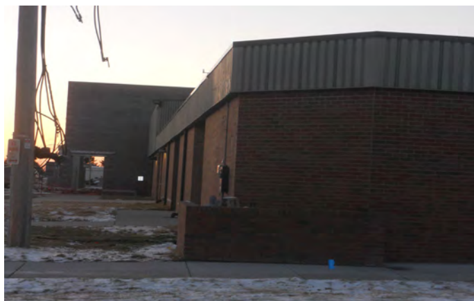
Four new classrooms are also being added to West Indianola.
