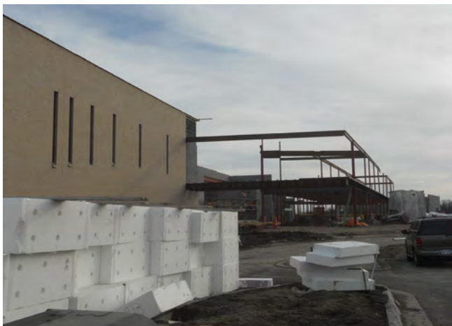
Middle school classrooms are being finalized.
