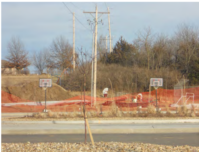
Seven new classroom additions to Elmont are nearing completion deadline.
